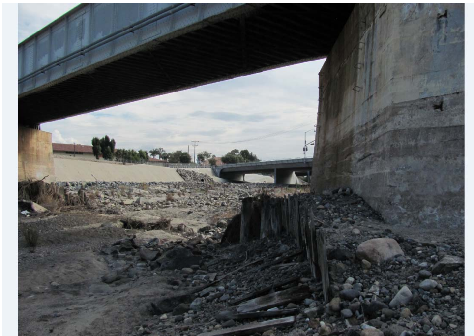
Figure 1 – San Juan Creek Bridge Pier (looking upstream)
